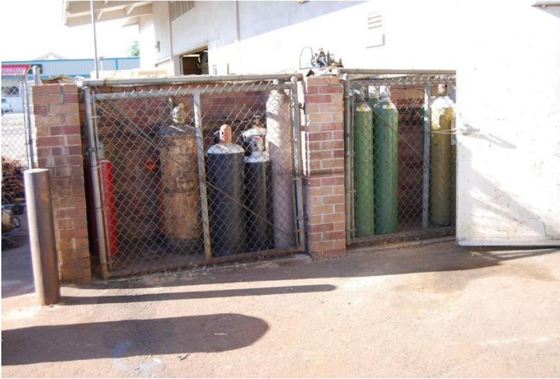
Gas storage – Cylinders should be clearly marked. Oxygen must be separated from fuel.
