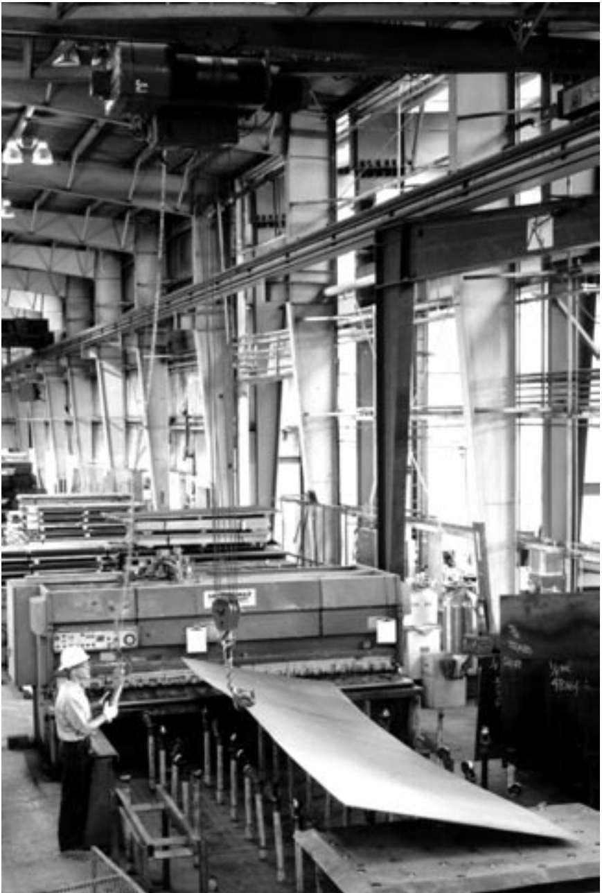
Laying Down A Sheet For The Shear
