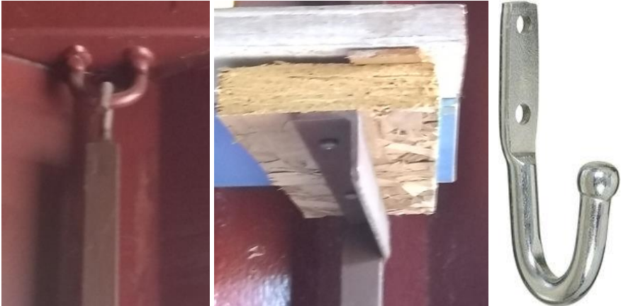
Brackets installed using a purchased hook.
